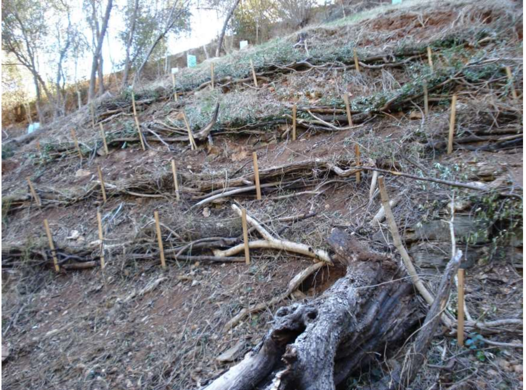
Using cut woody material to protect slopes
